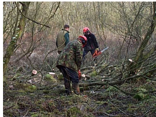
Work in progress in the New Forest
