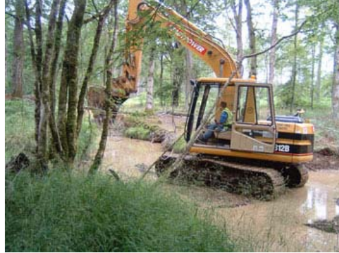
Work in progress in the New Forest
